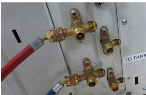
Installation of rubber hose
